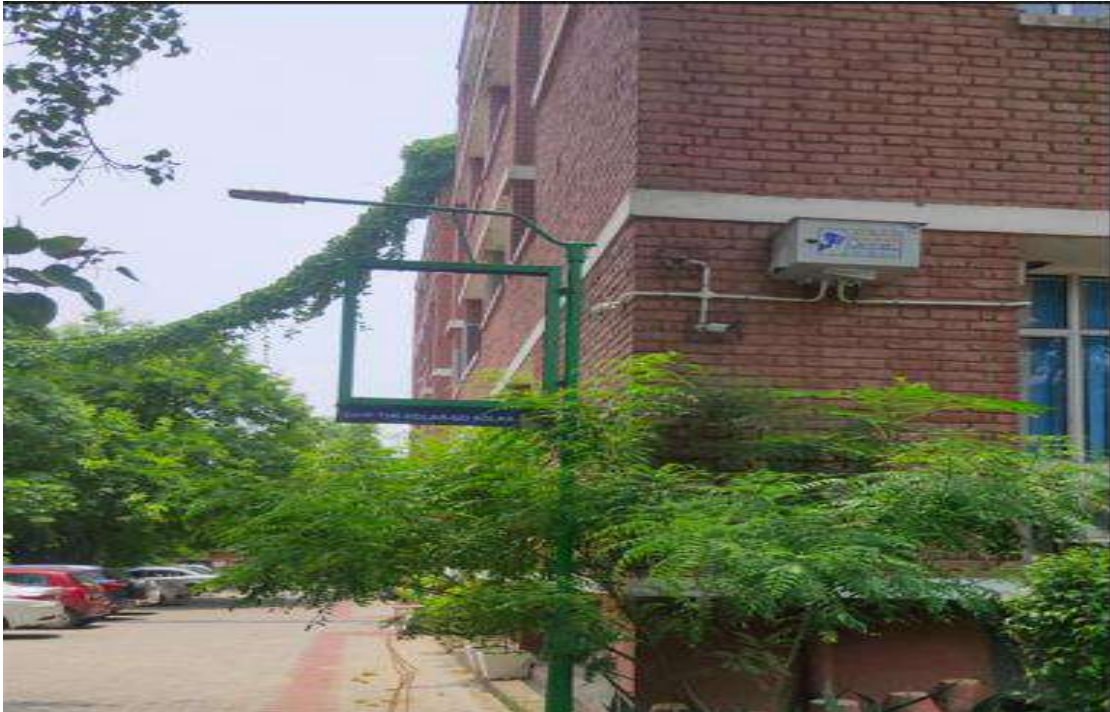
Figure 21: Site Photograph – Solar Street Light
