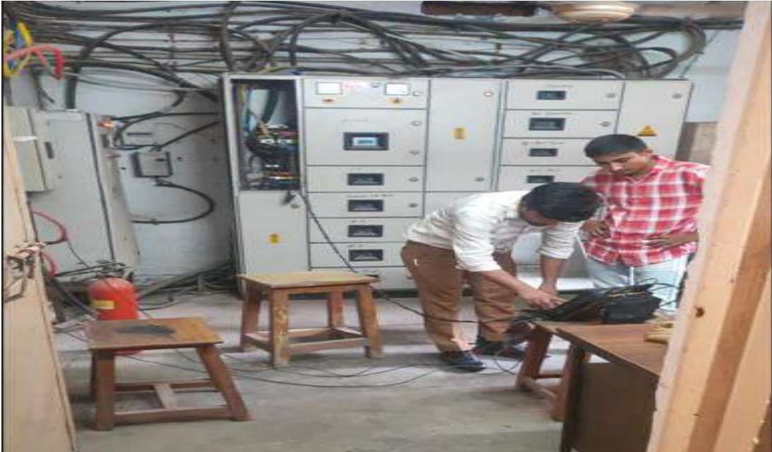
Figure 19: Site Photograph 1 – Energy Recording at Main Incomer
